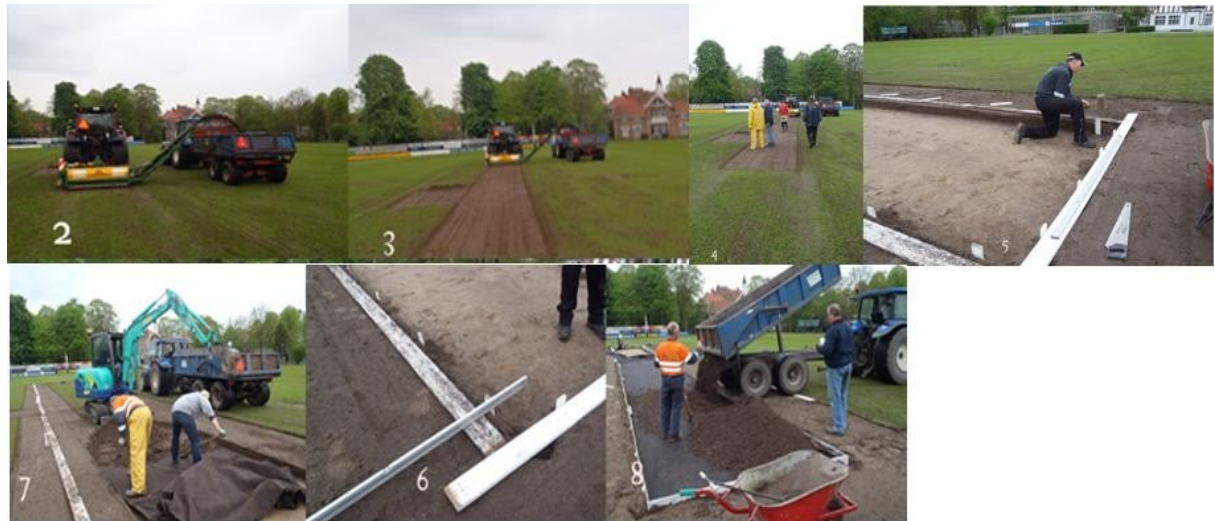
Figure 4.1.2. Excavation of a cricket pitch
